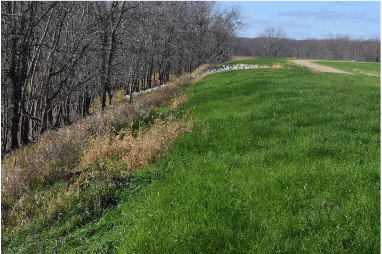
South exterior slope
