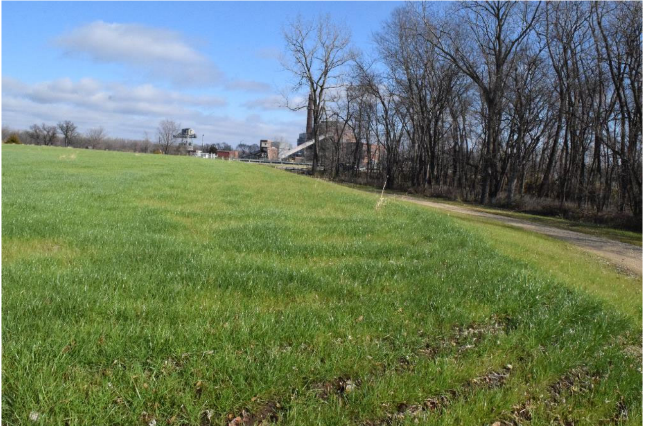
South exterior slope
